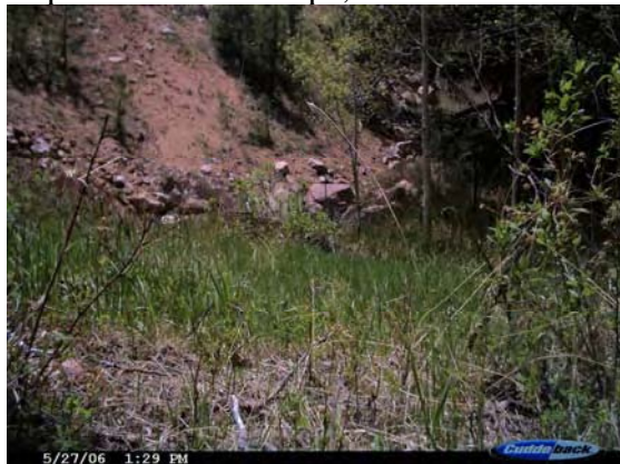
Impact Site 1: fill slope, west side
