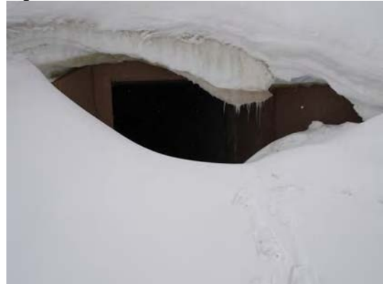
April 2006 (west side)
