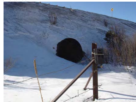
Control Site 2: Roland Gulch culvert, west entrance
