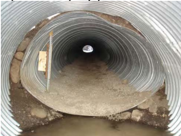
Impact Site 3: temporary lynx structure
