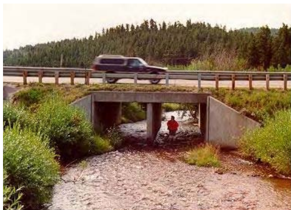
Control Site 1: Deer Creek span bridge 1
