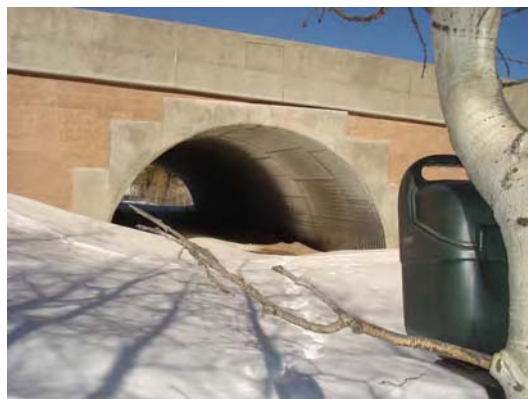
Impact Site 2 after construction
