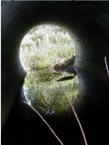
Impact Site 3: Long Hollow culvert 2
