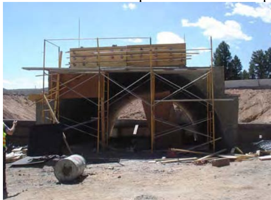
Impact Site 2 during construction of the southbound U.S. 285 portion of the underpass
