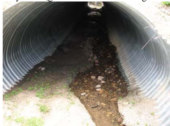
May 2006 (ground water flow through tunnel)
