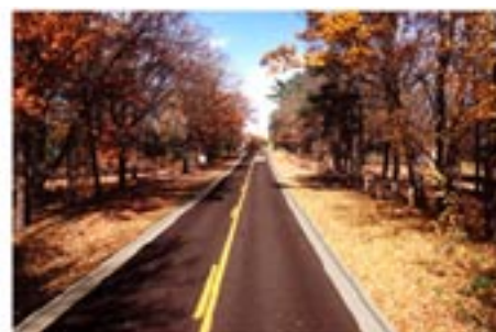
Urban Section - 11' Lane w/ Curb & Gutter
