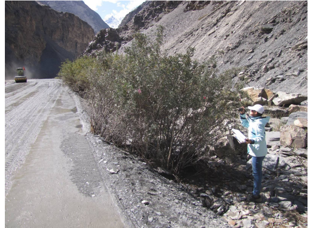
Fig 2. Roadside vegetation was protected entirely by modifying the highway cross-section designs and optimizing construction regimes (kilometer markers K757+550 along KKH in KNP, a is before KKH improvement project, b is after)
