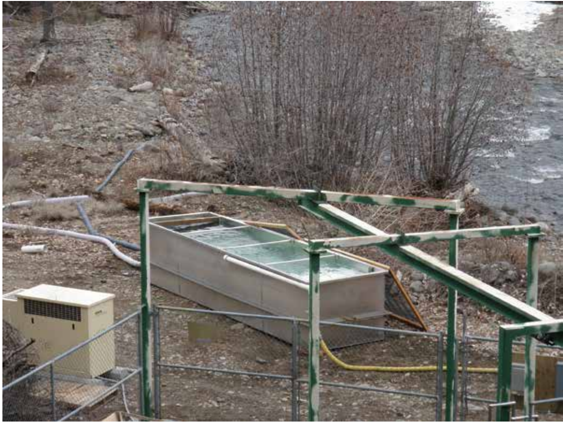
Photograph 1. Mobile Coho Salmon acclimation tank installed along Rattlesnake Creek, tributary to the Naches River in the Yakima River subbasin. Photo credit: Todd Newsome.
