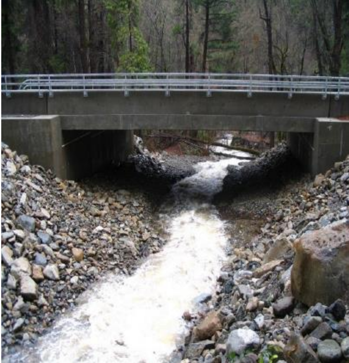
Figure 11: A properly sized bridge for fish passage that does not constrict water flow or channel migration. Image courtesy of Caltrans.
