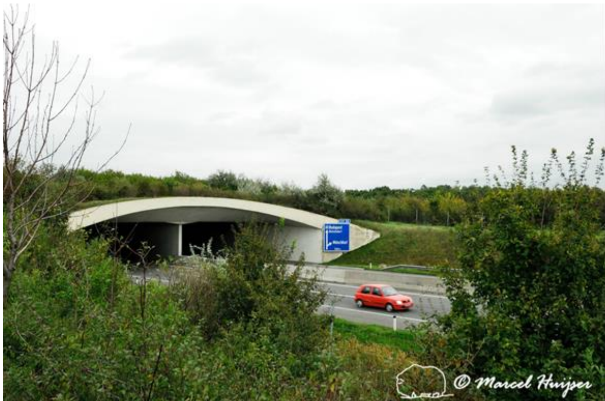
Figure 5: Multifunctional overpass (wildlife and farm road), about 100 meters wide, across A4 motorway, Parndorf, Austria. The overpass is designed for farmers, agricultural machinery, hunters and wildlife including
