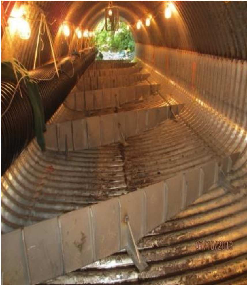
Figure 6: Fish passage structure. Photo courtesy of Caltrans.
