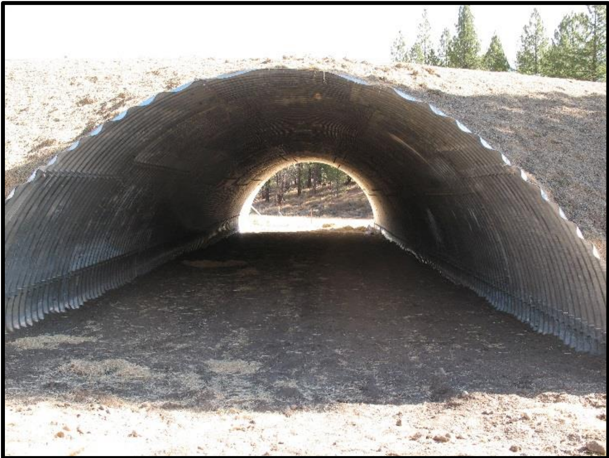
Figure 14: Wildlife underpass on US Highway 89 in the Sierra foothills. Photo courtesy of Suzanne Melim, Caltrans.
