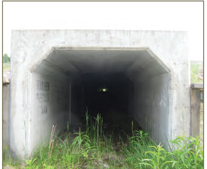
Photo 4. Open-bottom tunnel along highway 69, Ontario. © K. Gunson
