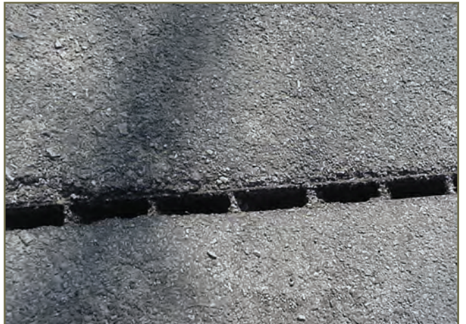
Photo 17. Zoom-in of open-top pipe culvert at road for Timber Rattlesnakes in Illinois, U.S. © S. Ballard
