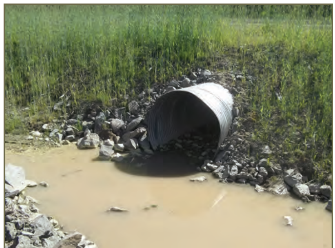
Photo 46. Pooling at culvert entrance that should be avoided at terrestrial wildlife tunnels © K. Gunson
