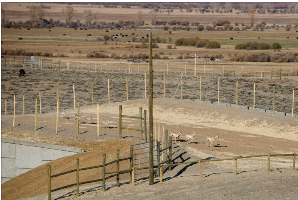
Figure 12—Pronghorn antelope using overpasses at Trappers Point near Pinedale, Wyoming.
