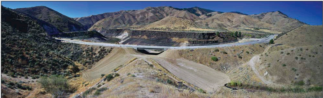
Figure 3— Idaho State 21 wildlife underpass.
