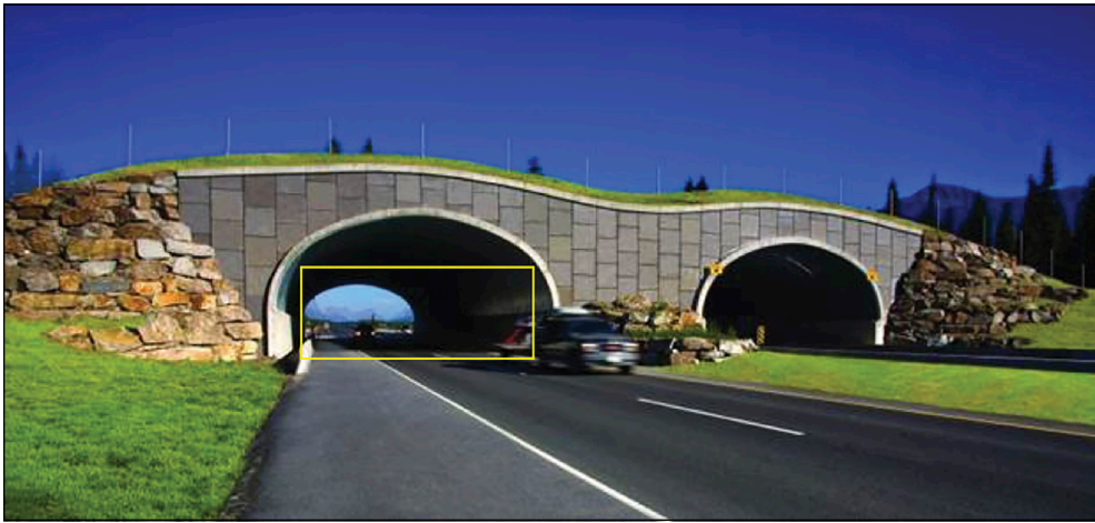
Figure 6—Two-span wildlife crossing over Trans-Canada Highway in Banff National Park, Alberta, Canada (the yellow box depicts the clearance box).
