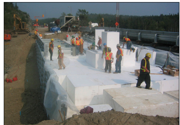
Figure 13—Expanded poly-styrene geofoam used in construction.
