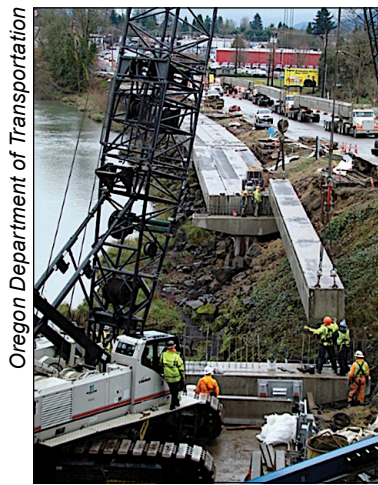
Figure 8—Crews place large concrete box beams for the new path viaduct near the Willamette River in Oregon.
