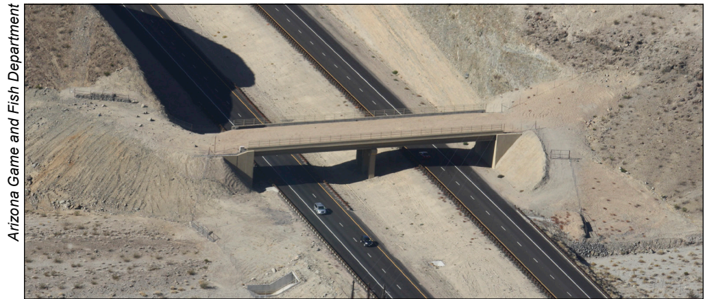
Figure 4—Traditional bridge-style wildlife overpass crossing on U.S. Highway 93 in Lake Mead National Recreation Area to protect desert bighorn sheep.
