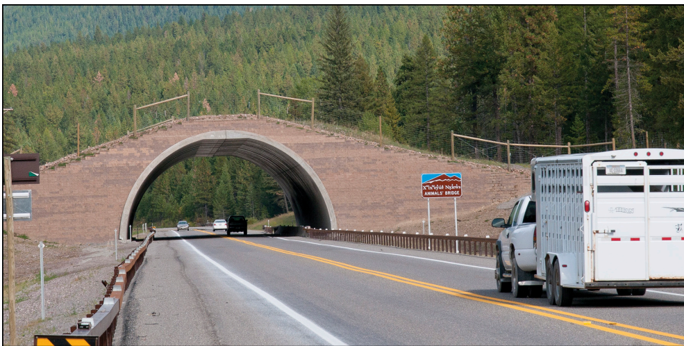
Figure 7—Single-span wildlife crossing known as the “Animals’ Trail,” a 197-foot wide vegetated arch overpass for wildlife that crosses over U.S. 93 on the Flathead Indian Reservation, home to the Confederated Salish and Kootenai Tribes.
