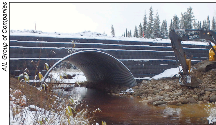
Figure 12—Geosynthetic reinforced soil is used for a buried bridge during construction.
