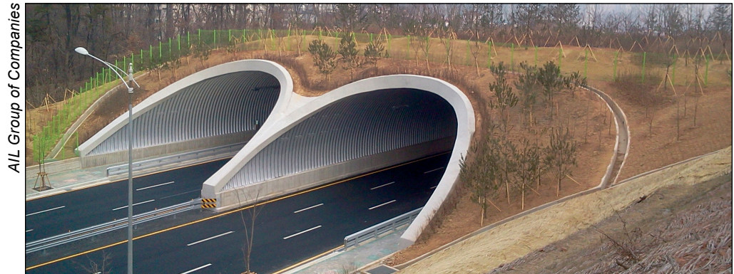
Figure 11—Bevel end treatment on Nambu Beltway Tunnel in Gyeonggi Province, South Korea.
