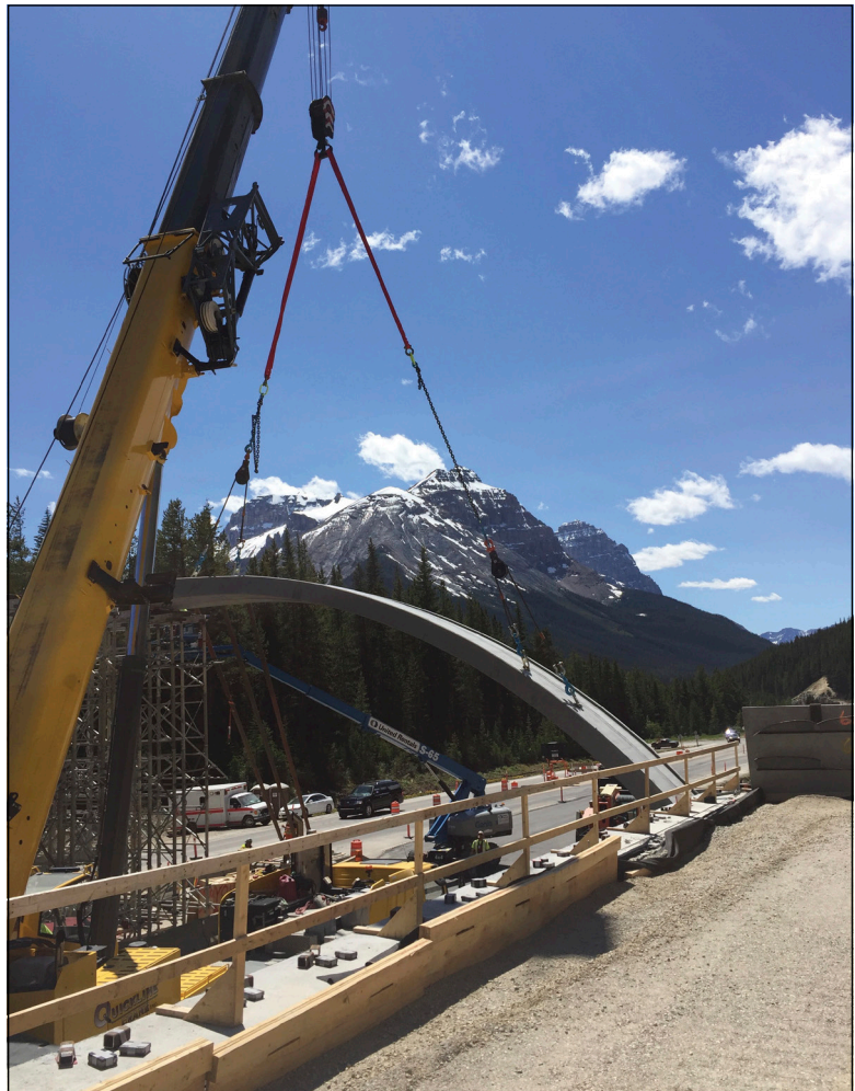
Figure 14—Cranes erecting concrete arches over the Trans-Canada Highway in Yoho National Park.
