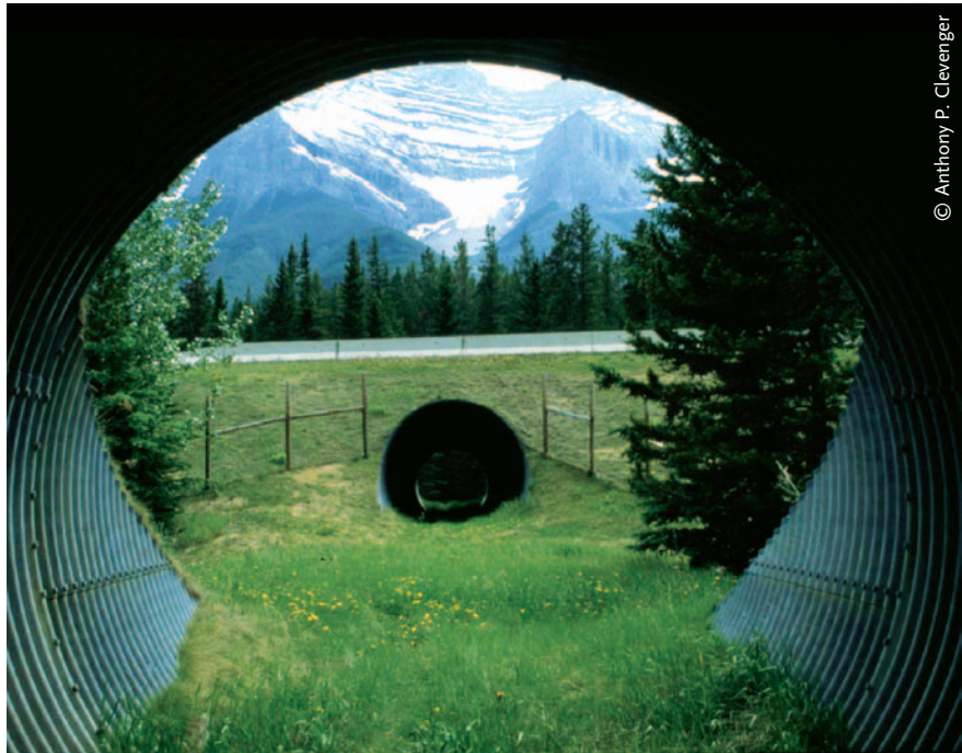
Metal culvert underpass, four meters in diameter and built in 1983.
