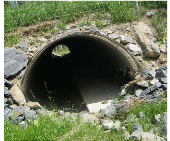
This culvert crossing on the Caribou Bypass includes a shelf to allow terrestrial animals to cross in wet conditions. (Courtesy of MaineDOT)
