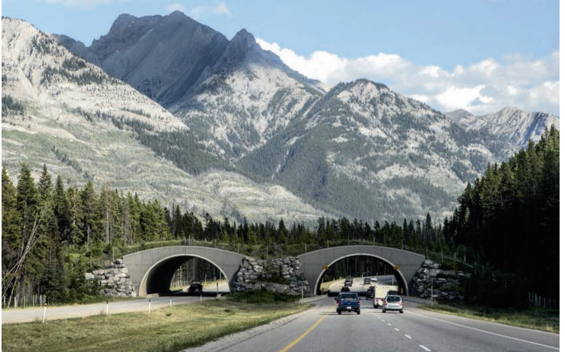
De Bourgeau Overpass, ecoduct over de Trans-Canada Highway in Banff National Park.
