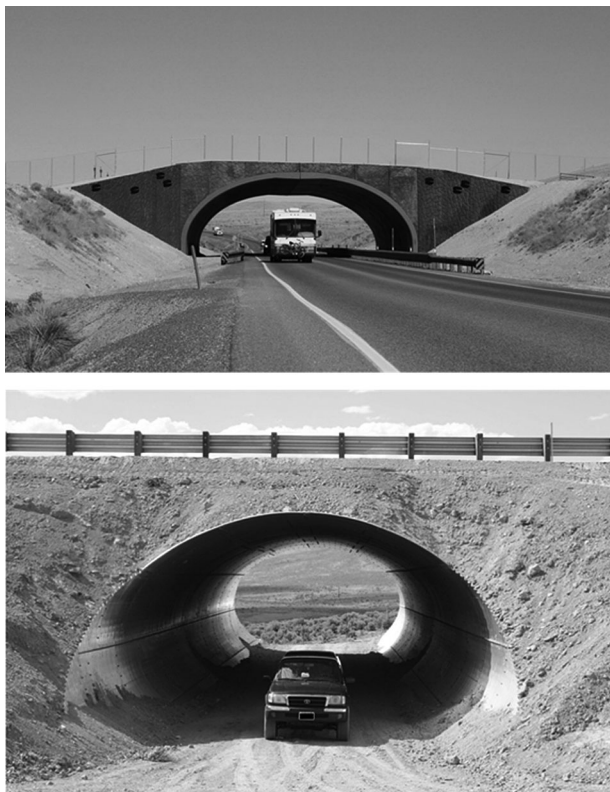
Figure 2. Examples of wildlife crossing structures: overpass (top), and underpass (bottom). We investigated structure use by migratory mule deer at 10-Mile and HD Summits on US 93 between Wells and Contact, Nevada, USA, 2010–2014. Each underpass was 8 m wide by 28 m long, and 6 m tall; the vehicle in the underpass is a 1999 Toyota Tacoma to provide a visual indicator of size of the structure.
