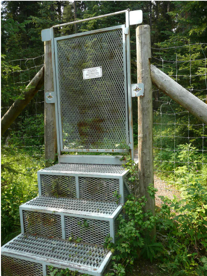
Step gate with spring-loaded door situated at trailhead in Banff National Park, Alberta (Photo: Tony Clevenger).
