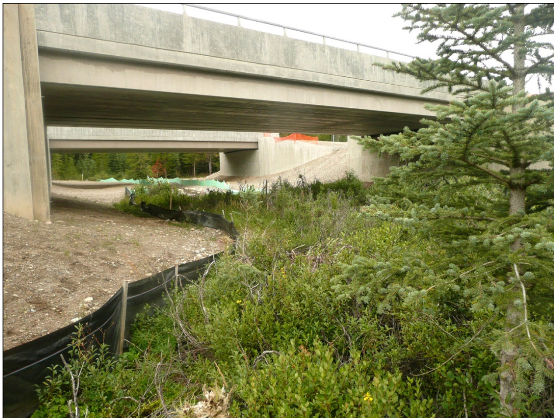
Wildlife underpass designed to accommodate water flow (Photo: Tony Clevenger).
