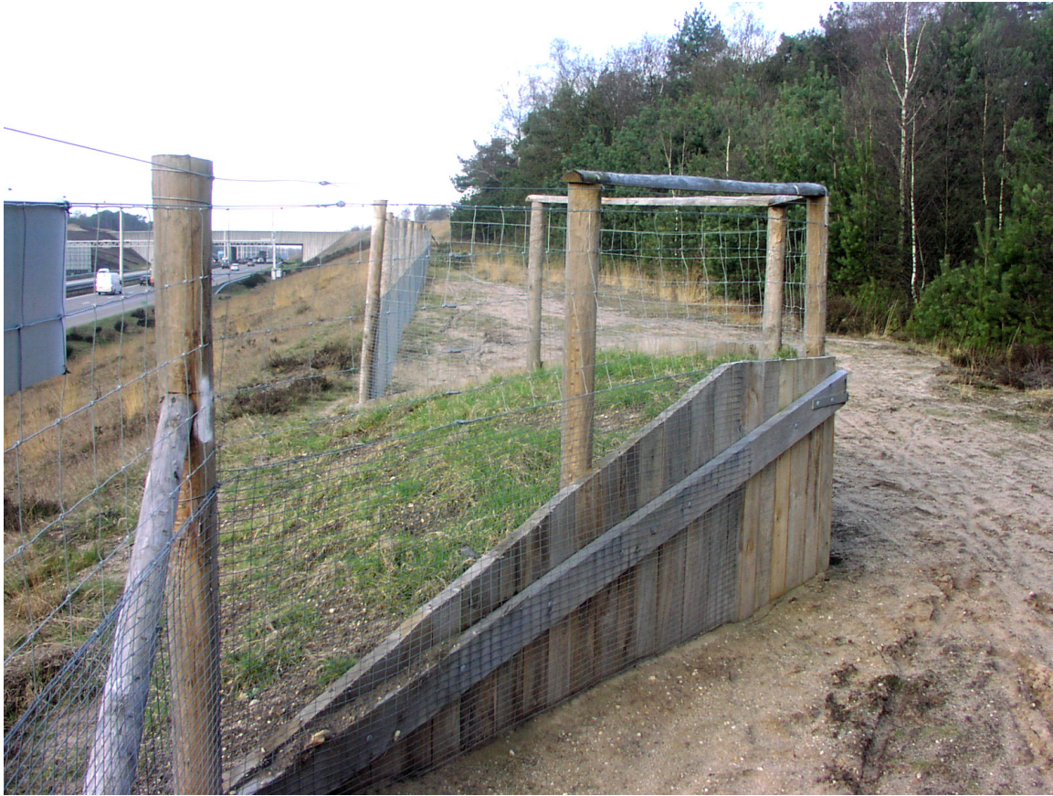
Wildlife "jump-out" escape ramp (Photo: Tony Clevenger).
